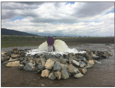
Full operation of pump system - Outlet Structure in Basin 2
