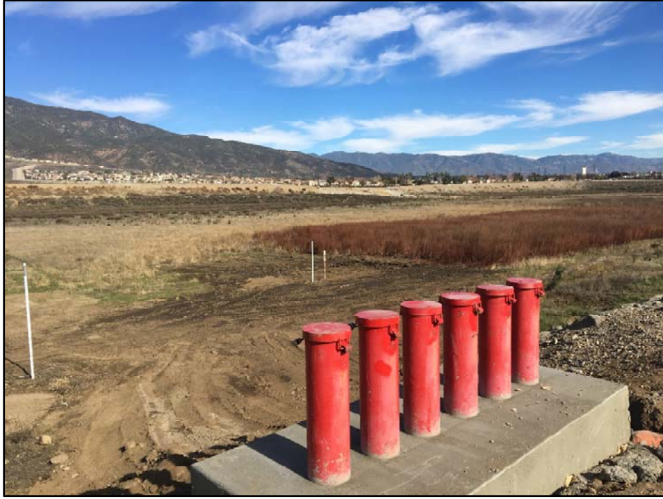
Completed Lysimeter System at Basin 2
