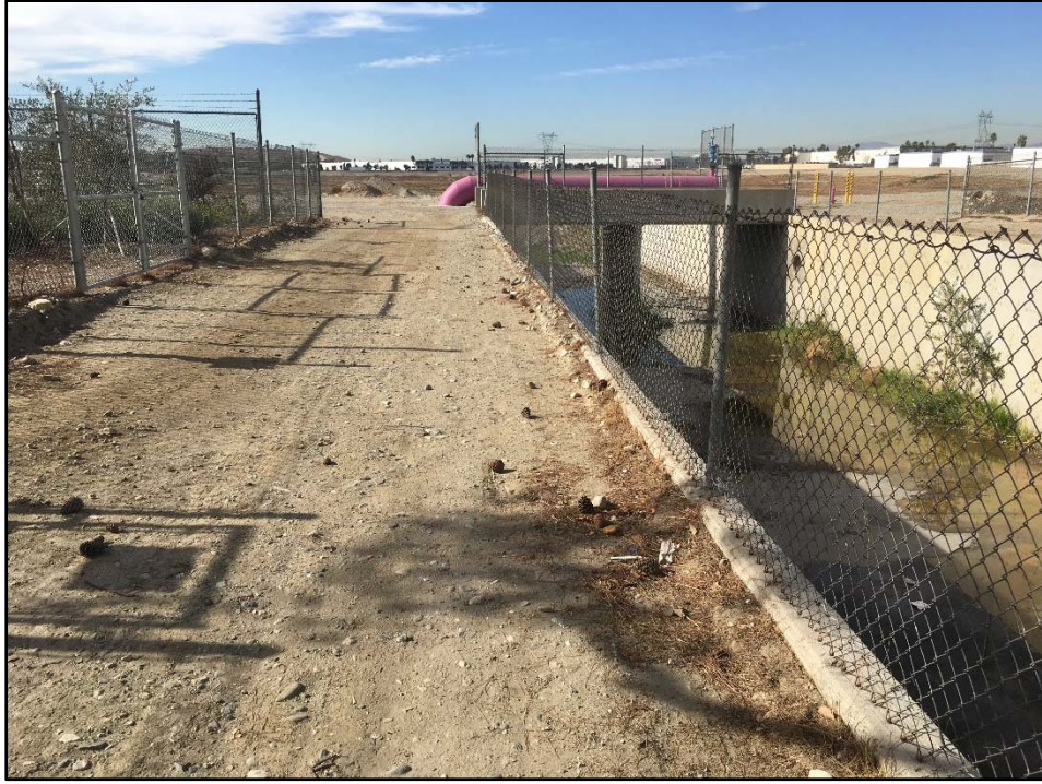
Near Wineville - Path of New 30-Inch Pipeline
