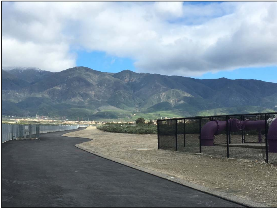
Completed RW Turnout
