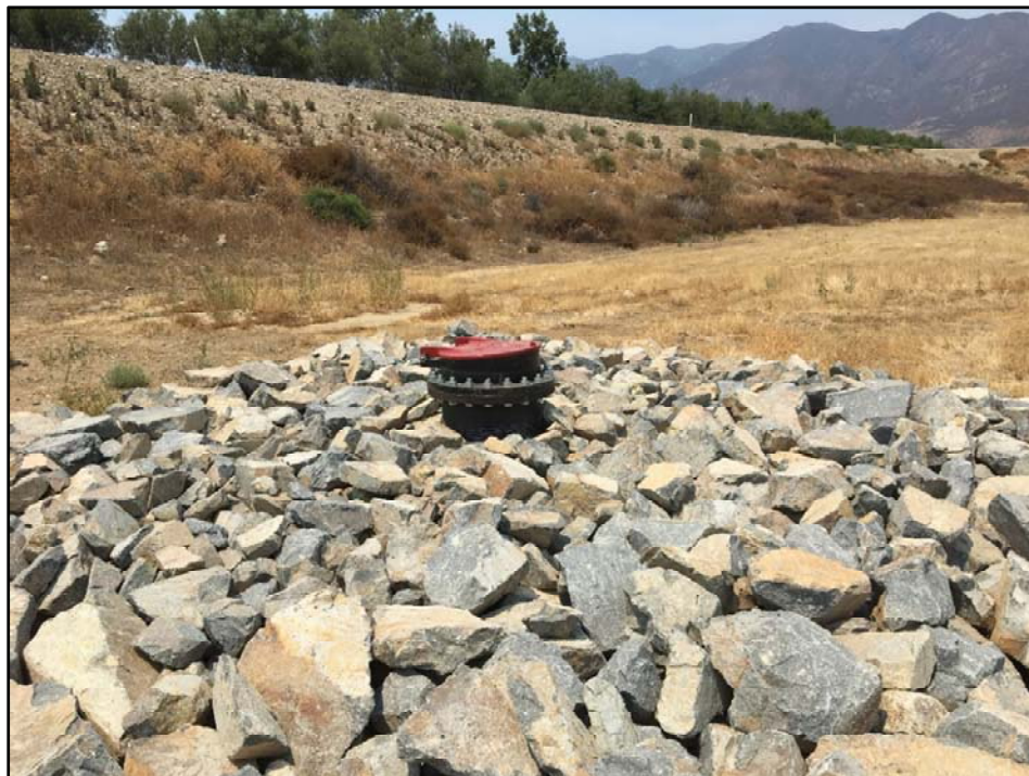
Completed Stormwater Outlet Structure in Basin 3
