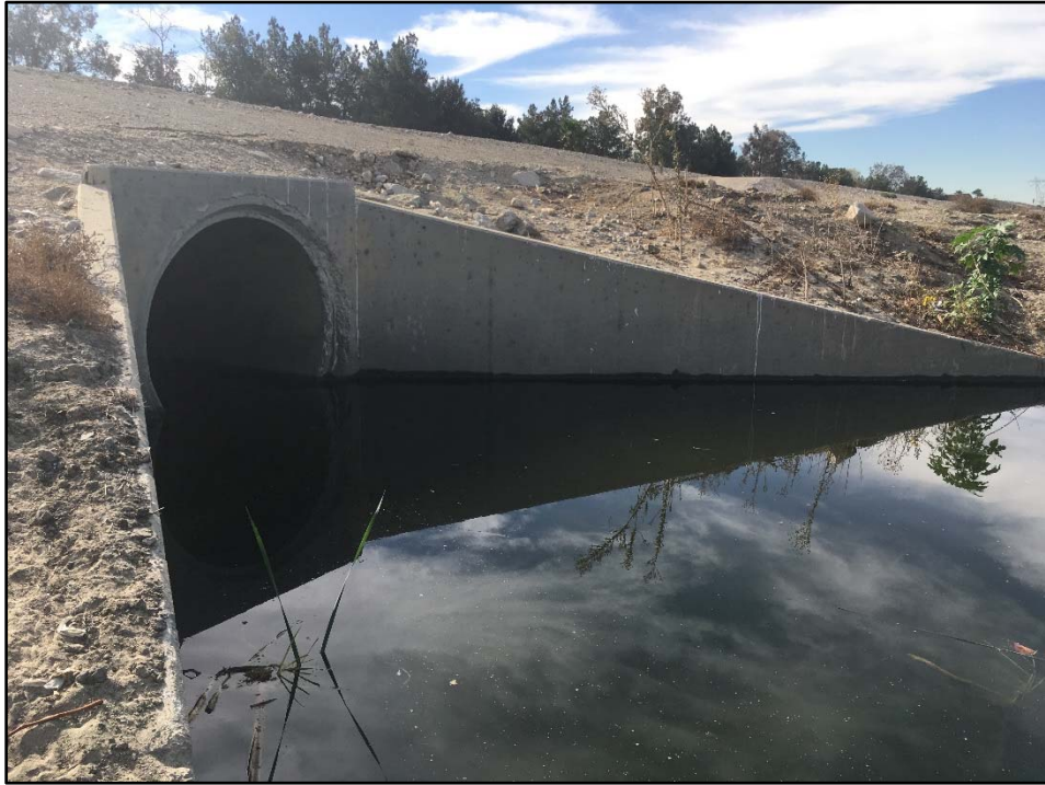
Wineville – Existing Basin Outlet
