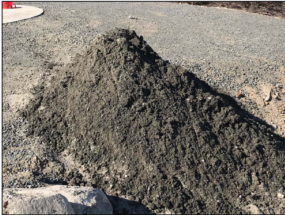
Removed Alluvial Deposits within the Pump Station Wet Well (less than 1 cubic yard)
