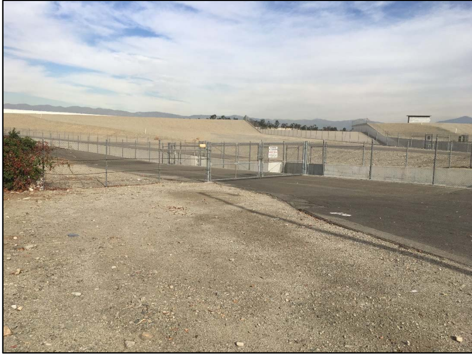
Near Jurupa Path of New 30-Inch Pipeline
