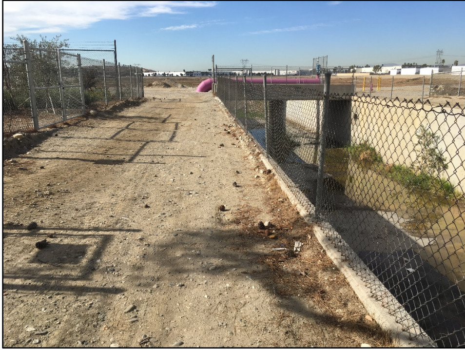
Near Wineville - Path of New 30-Inch Pipeline
