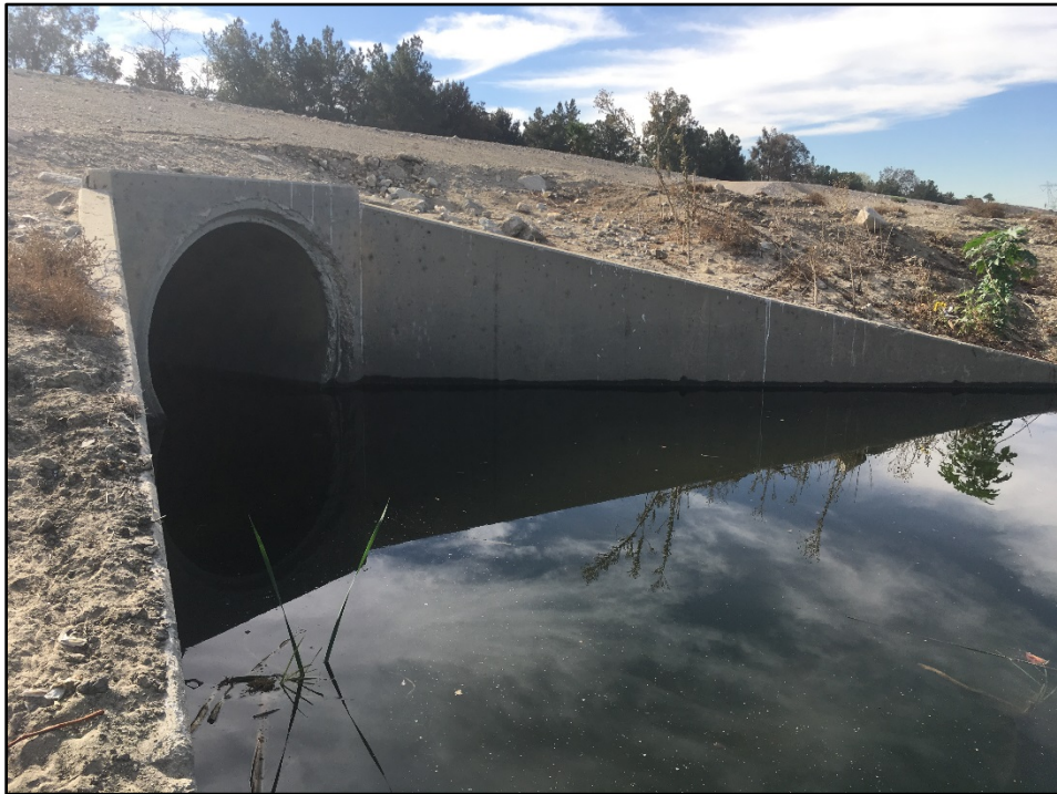
Wineville – Existing Basin Outlet
