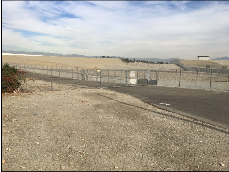
Near Jurupa Path of New 30-Inch Pipeline
