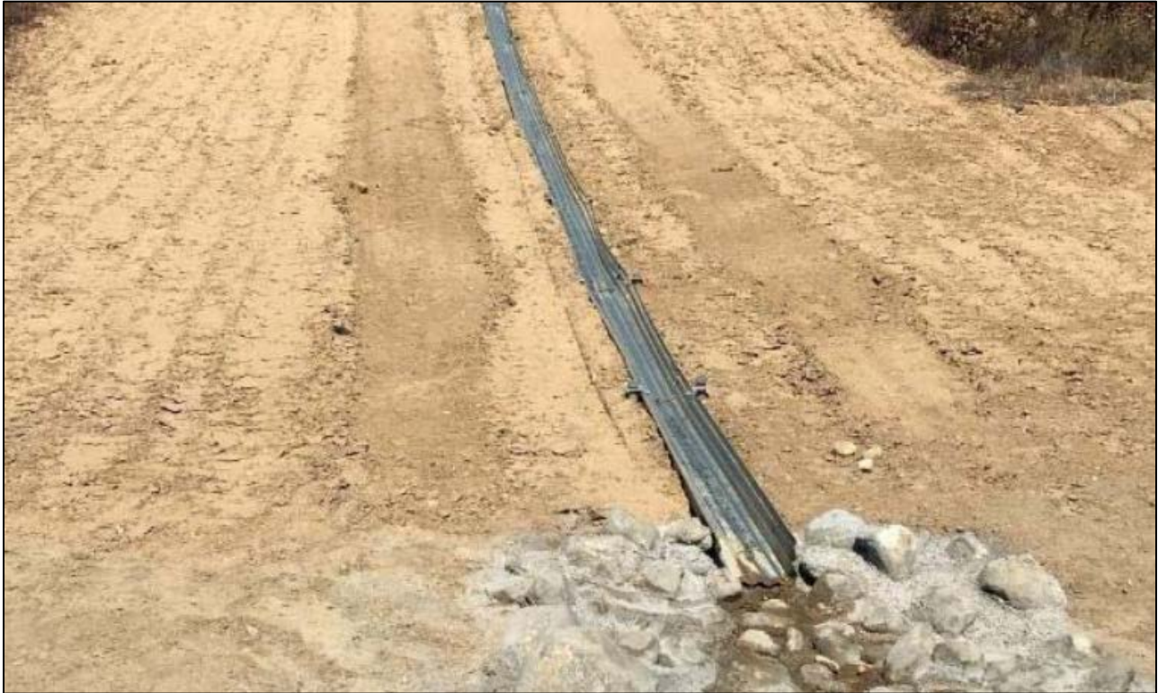
Lower Day – Added Down Drains to Minimize deposit into basin
