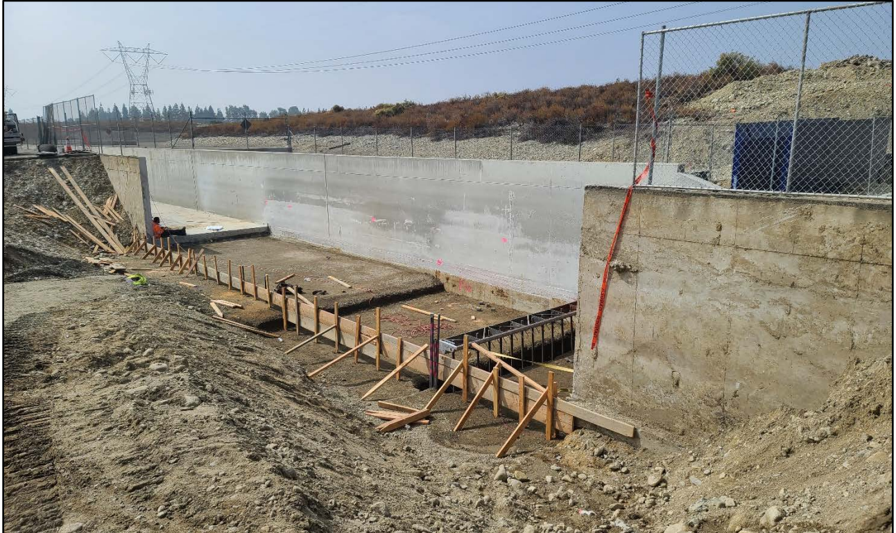
Lower Day – Demolished section of channel to prepare for new gate
