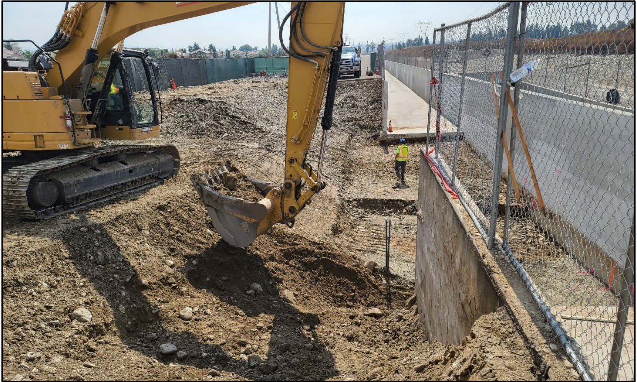
Lower Day – Construction at Channel
