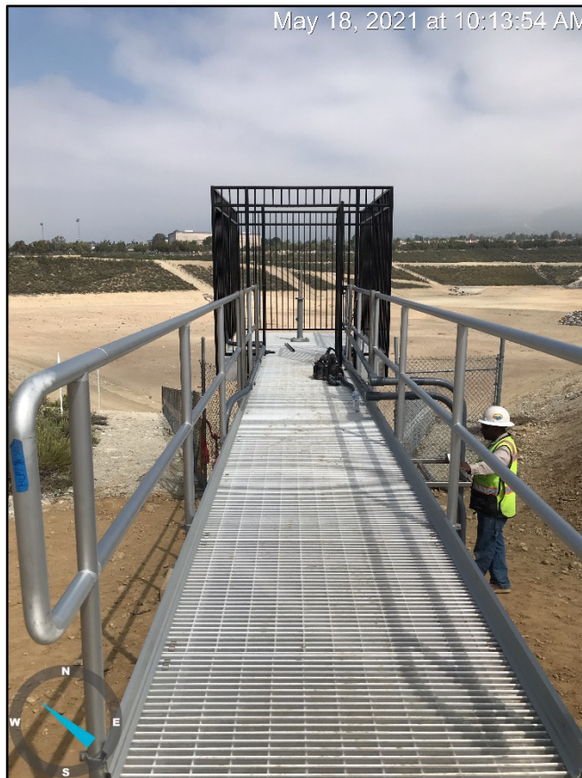
Lower Day – New Catwalk for Cell 3
