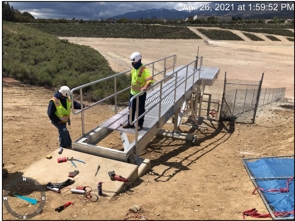
Lower Day – New Catwalk for Cell 3
