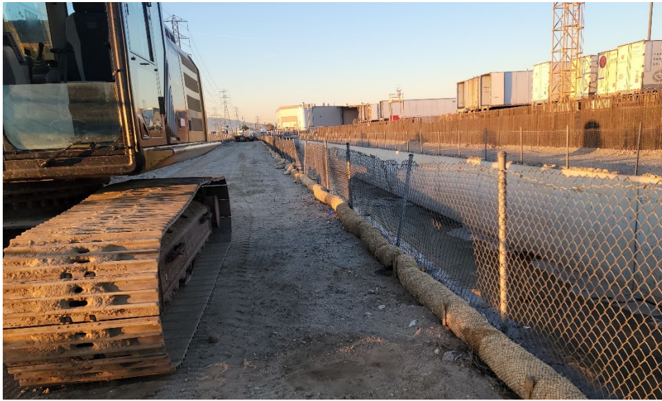
Wineville/Jurupa Storm Water Distribution Pipeline (Construct along Etiwanda Channel)
