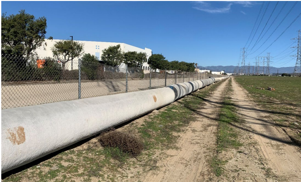
Wineville/Jurupa Storm Water Distribution Pipeline (Received Pipes)
