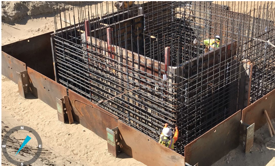
Wineville/Jurupa Storm Water Distribution Pipeline (Wet Well Construction)
