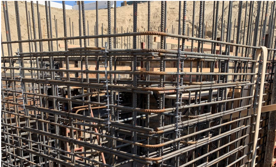
Wineville/Jurupa Storm Water Distribution Pipeline (Rebar Work)
