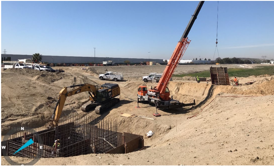
Wineville/Jurupa Storm Water Distribution Pipeline (Wet Well Shoring)
