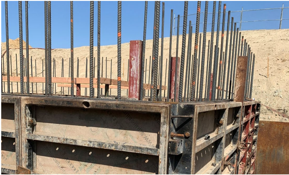
Wineville/Jurupa Storm Water Distribution Pipeline (Placement of Concrete Forms)
