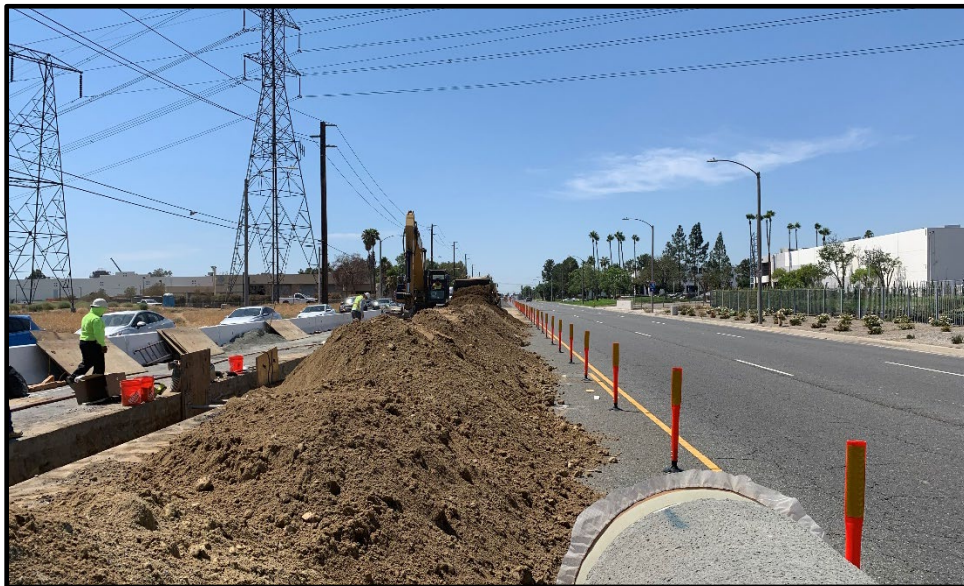
Wineville/Jurupa Storm Water Distribution Pipeline (Continued Construction Along Jurupa Street)
