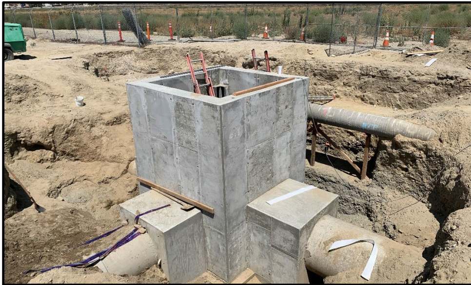
RP3 Basin Improvement (Construction of New Diversion Structure at RP3)
