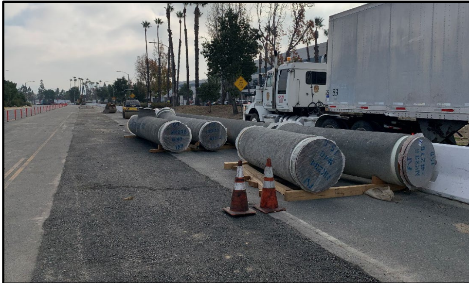
Wineville/Jurupa Storm Water Distribution Pipeline (Pipeline Construction on Jurupa Street)
