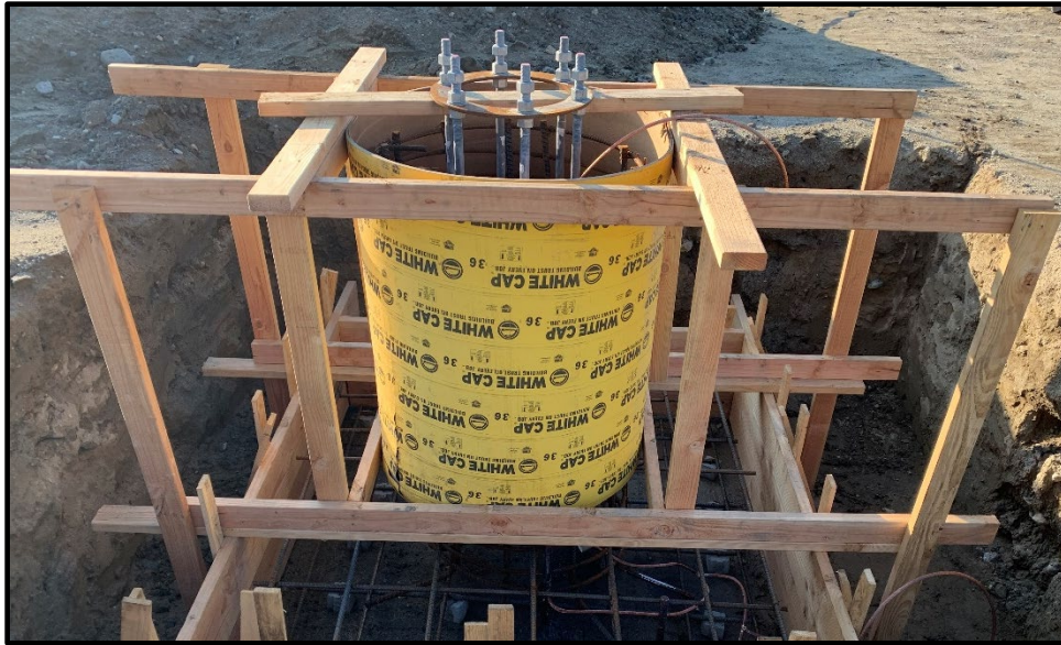
Wineville/Jurupa Storm Water Distribution Pipeline (Construction of the Monopole Foundation at Wineville)
