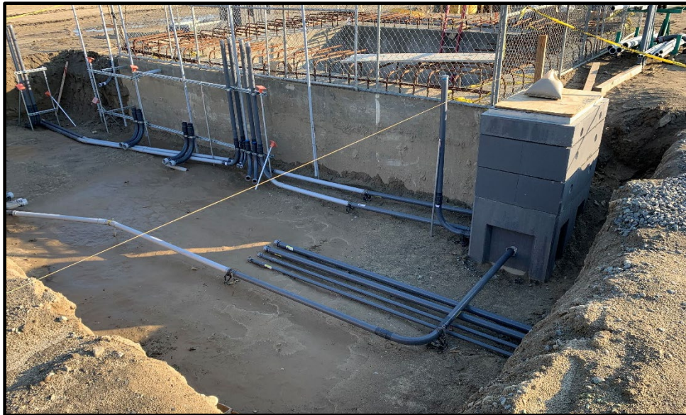
Wineville/Jurupa Storm Water Distribution Pipeline (Wet Well Construction Preparation of Slab with Underground Conduit)
