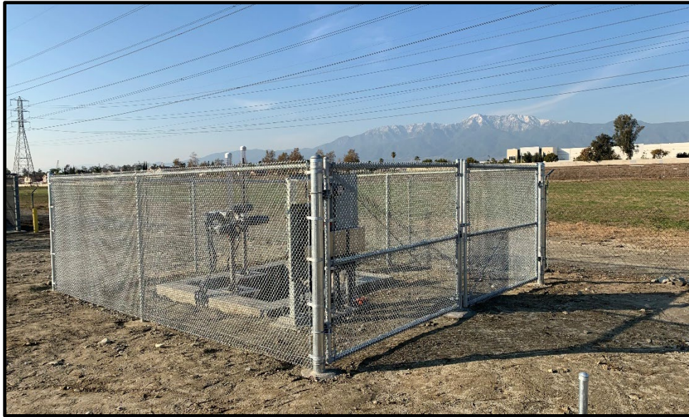
RP3 Basin Improvement (Completion of New Diversion Structure at RP3)
