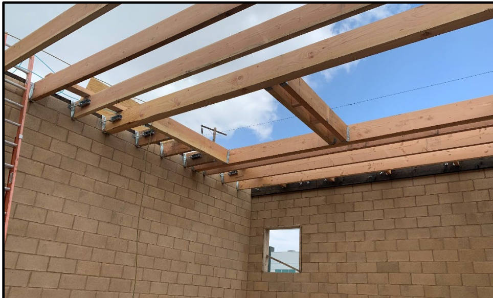
Wineville Basin – Pump Station (Joist Beams)
