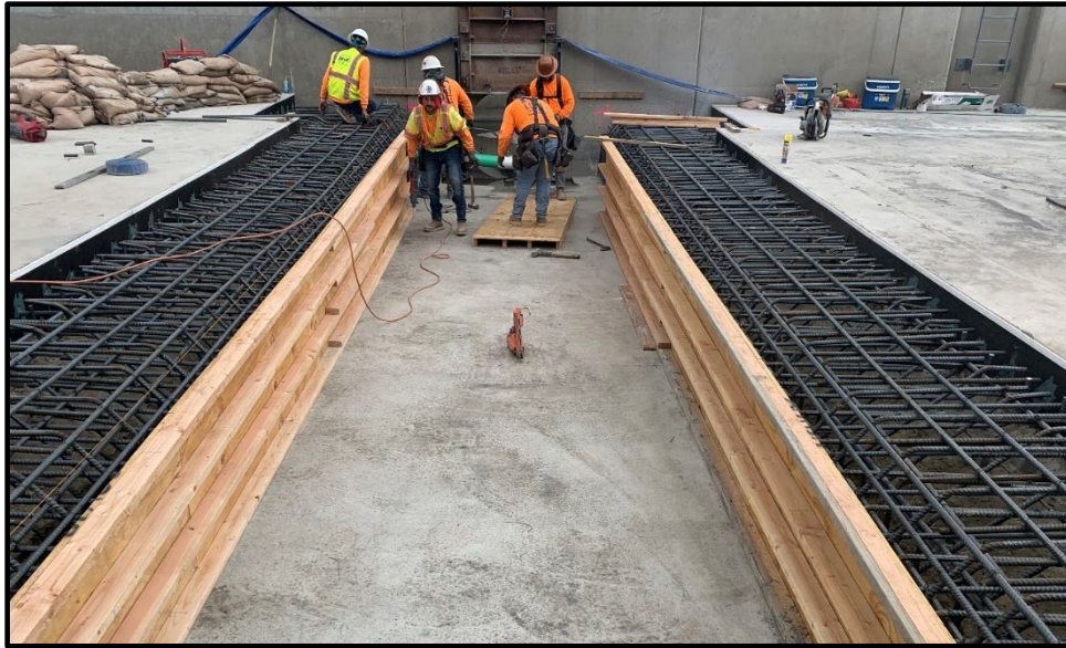
Jurupa Basin Improvement – Channel Diversion (Concrete work)
