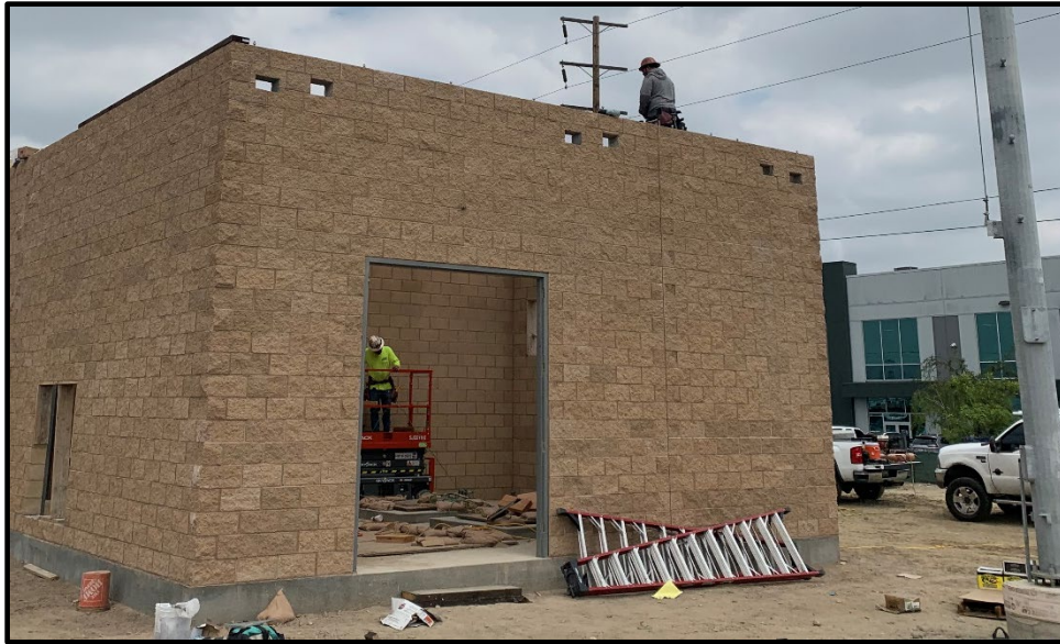
Wineville Basin – Pump Station Building South Side (Joist Beam Installation)
