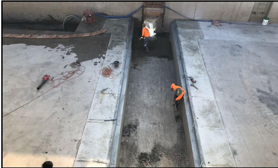
Jurupa Basin Improvement - Channel Diversion (Completed Concrete Work)
