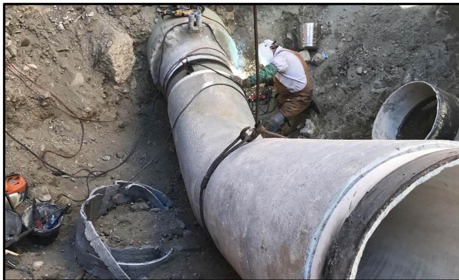
Jurupa Basin Improvement - Channel Diversion (Welding of New Piping into Jurupa)
