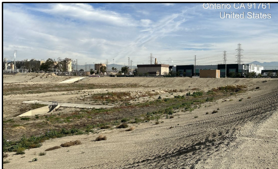
Wineville Basin Improvement – Basin (Completed Concrete Work in Basin)
