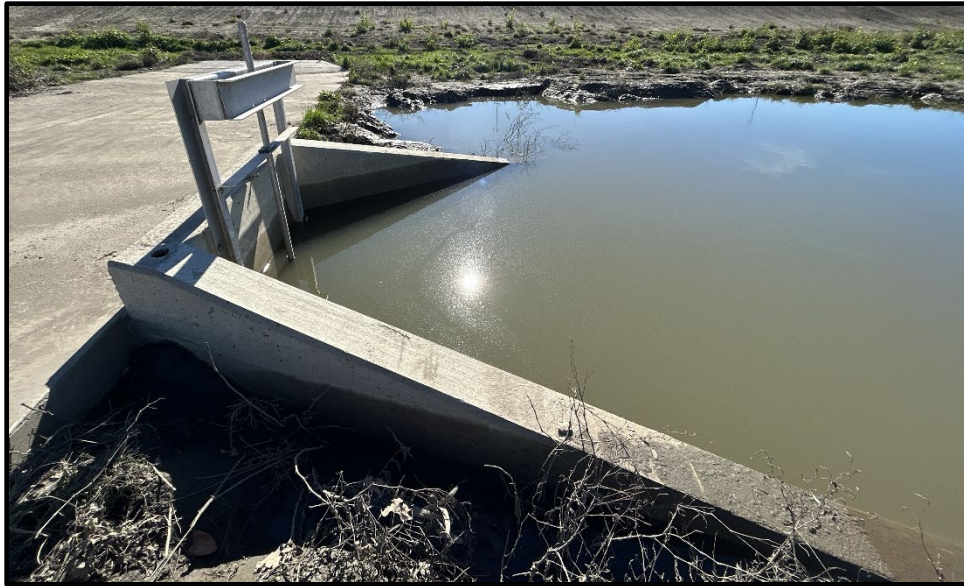
Wineville Basin – New Gate holding water before the Forebay Area (Completed Gate)
