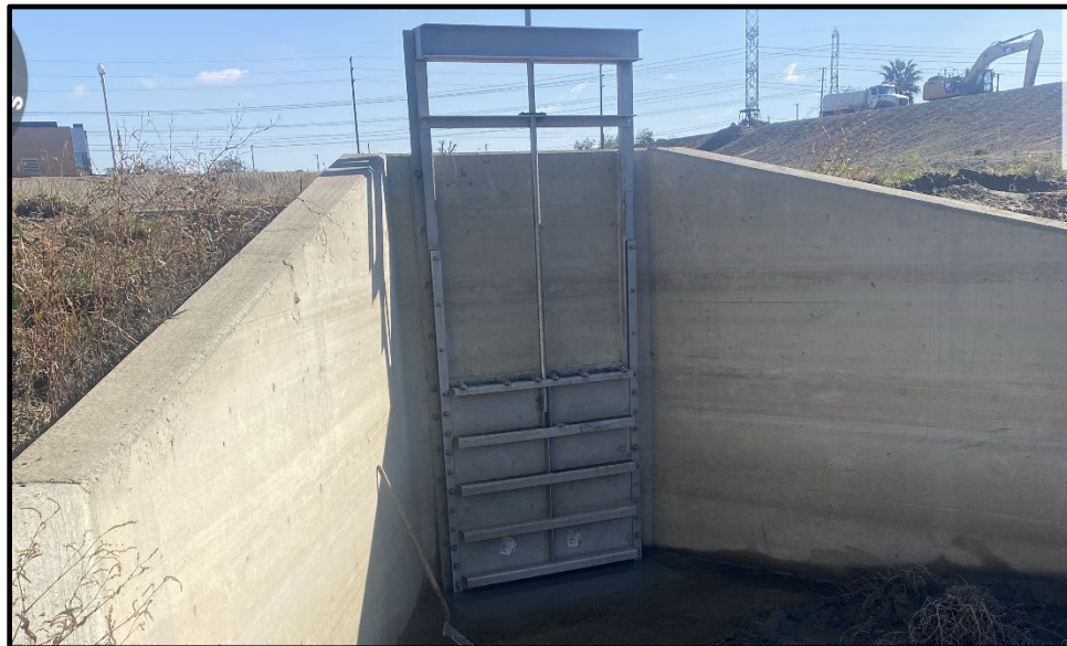
Wineville Basin Improvement – New Gate before the Forebay (Completed gate installation)
