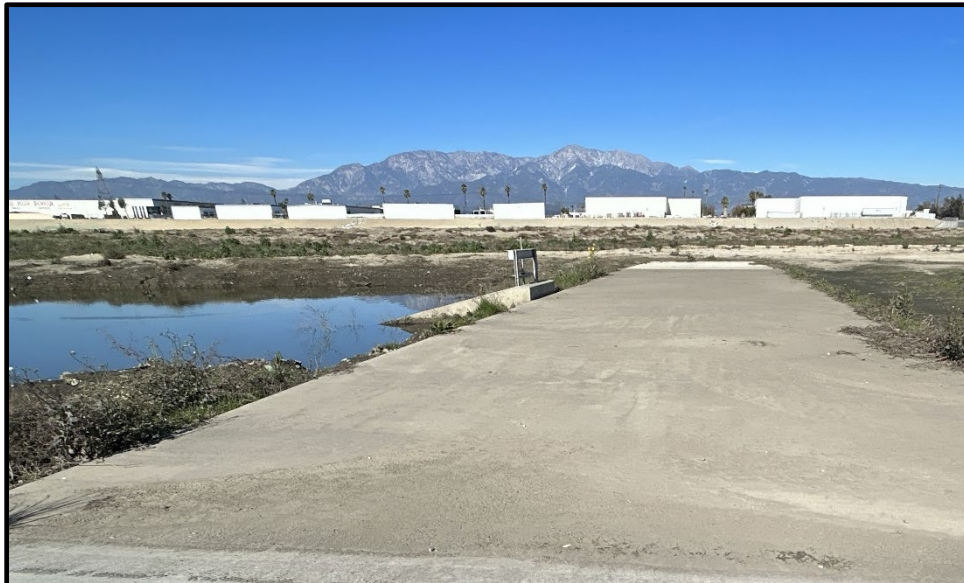
Wineville Basin – New Concrete to Forebay (Completed Spillway with New Gate)
