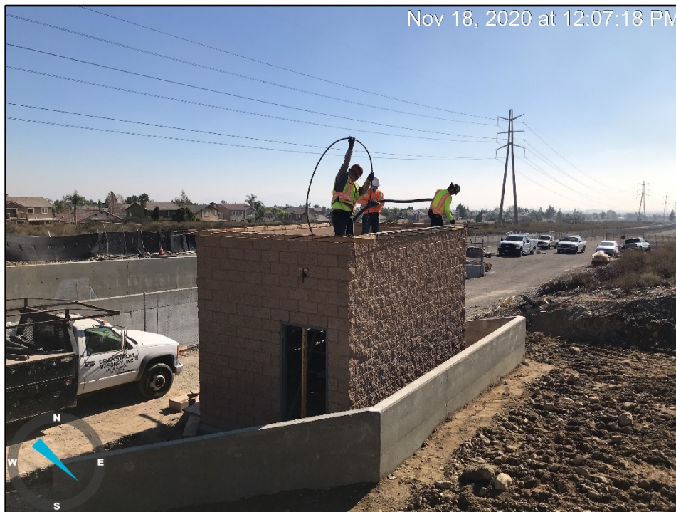
Lower Day – New Control Building
