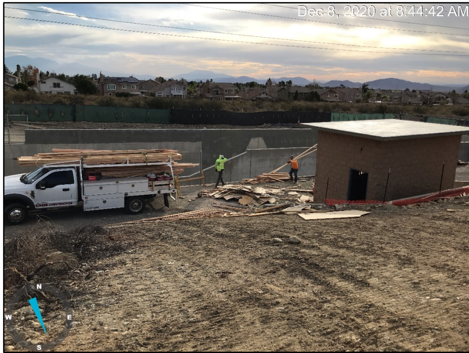
Lower Day – Completed Control Building
