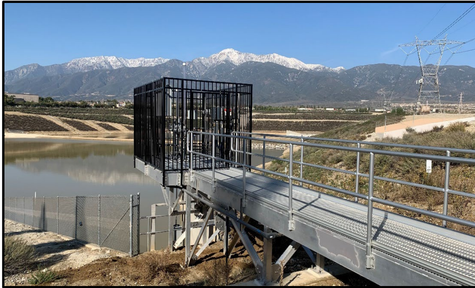
Lower Day Basin Improvement (Completed Catwalk Platform for new gates and level sensors at Cell 3)
