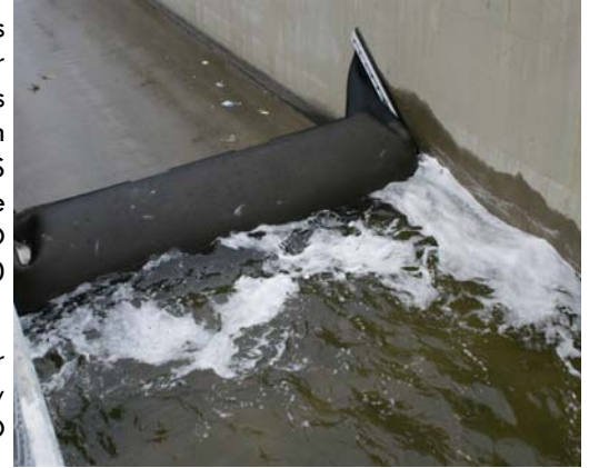
Rubber Dam in action
