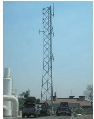
New Radio Antenna for the SCADA system
