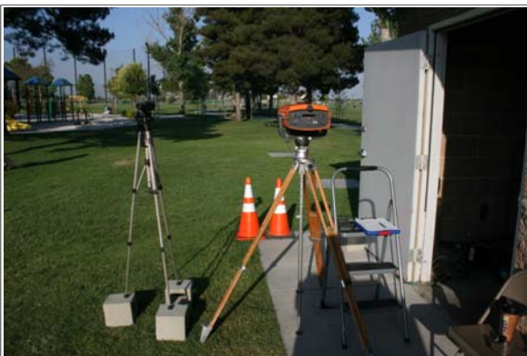
MZ-1 Monument Construction & Surveying
