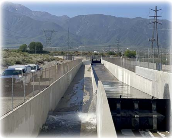
Newly Built Dam to Redirect Water Flow for Capture
