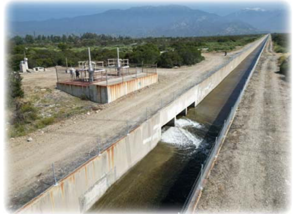
DYY Water Being Discharged to be Captured at a Basin
